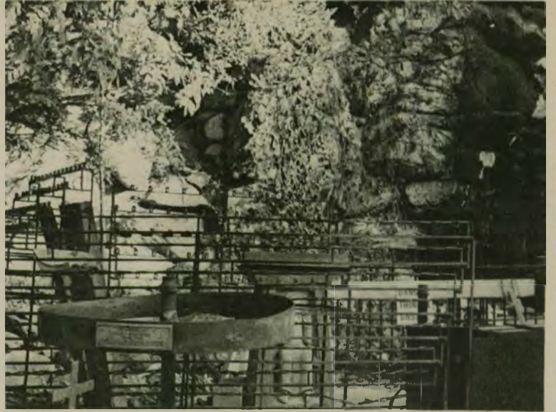
Reconstruction of the fire-damaged Grotto began almost immediately after the fire Monday. Story at left.
