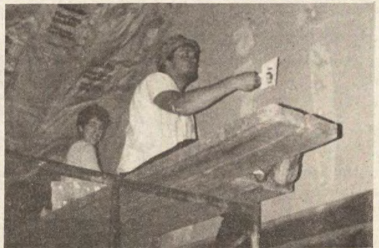
Students help to construct a dry wall
