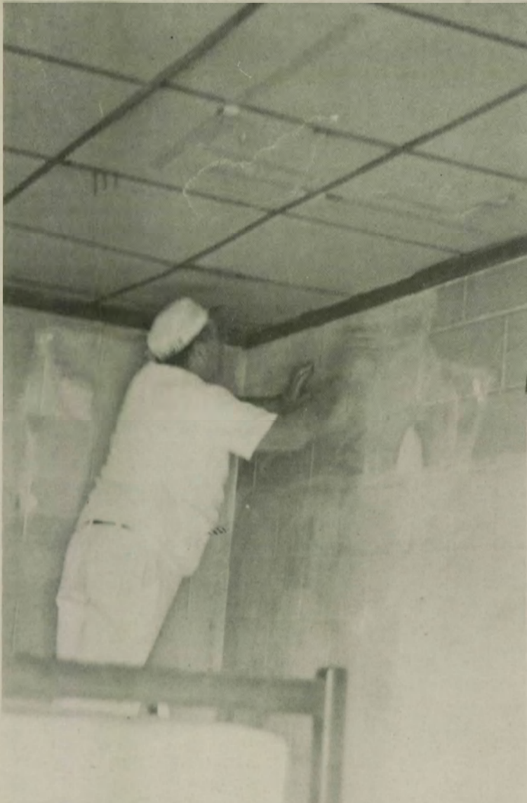
Repairs were started after a fire in Saint Mary's McCandless Hall Monday morning. The damage, estimated to be close to $2000, was caused by a faulty hotpot. Story on page 1.
