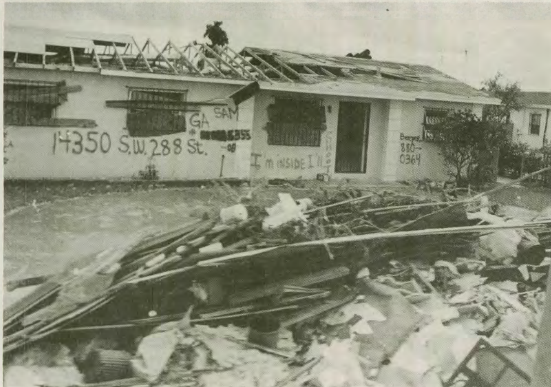
Many of the homes Goulds Park are still in need of repair
