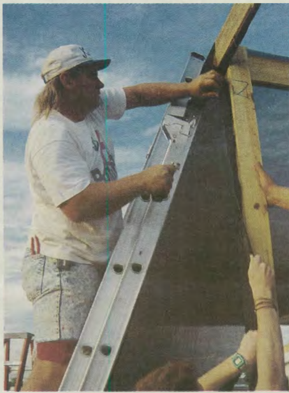
Craig Oliphant works to rebuild Florida homes. Oliphant organizes groups of volunteer workers to continue the relief effort in devastated areas.
