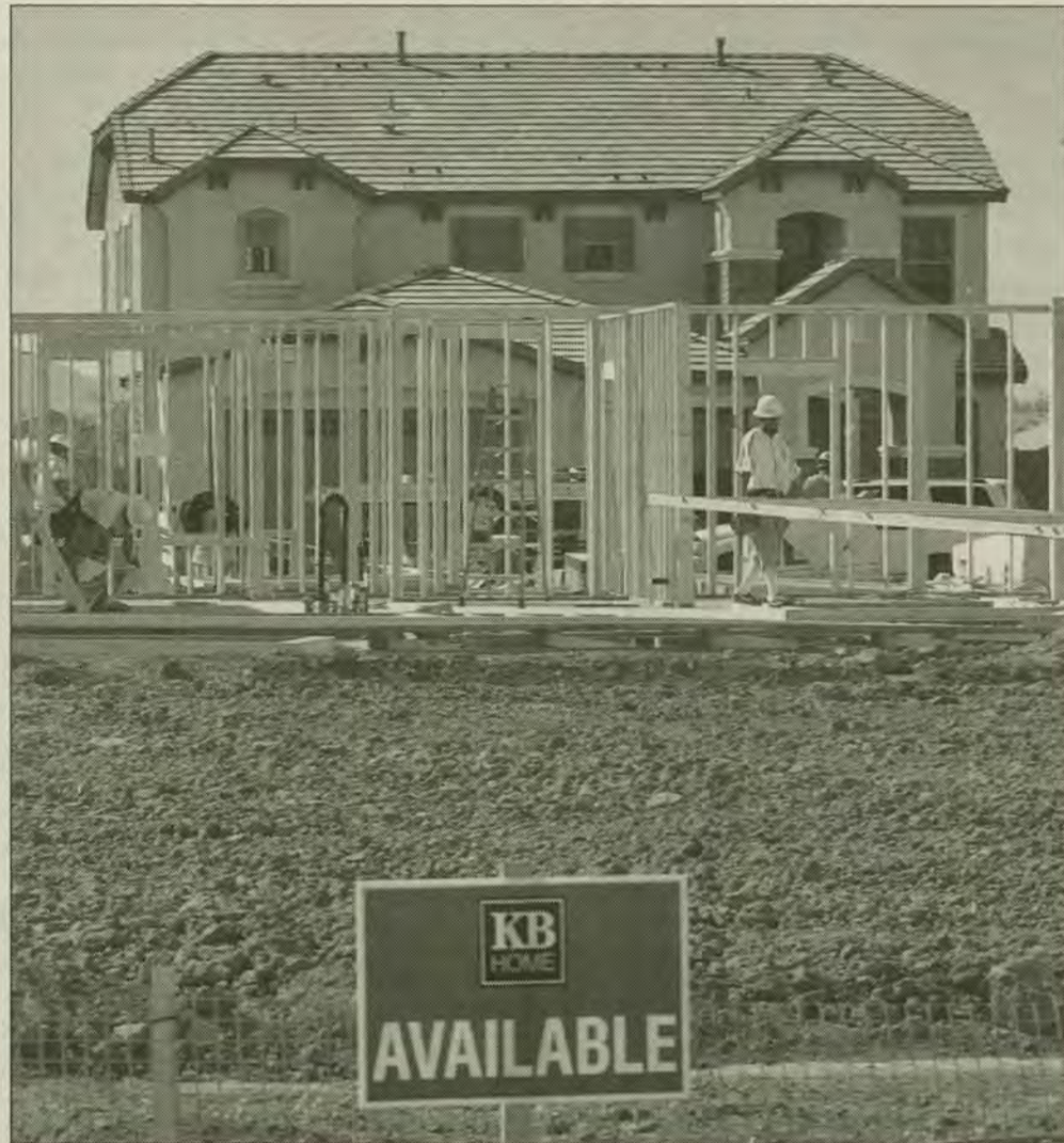
Workers build a new KB Home, one of the nation's largest home builders, in Gilbert, Ariz., Monday. KB Home said first-quarter fiscal earnings plunged in a housing slump.
