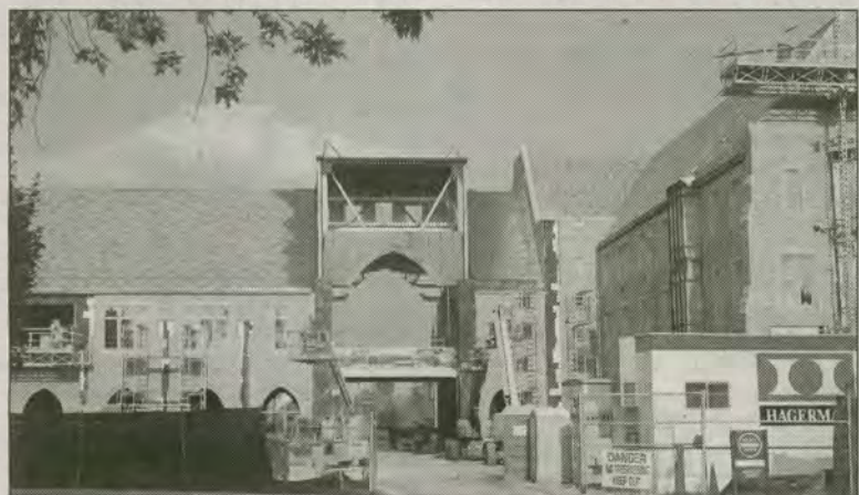
JESSICA LEE/The Observer The $57.7 million Eck Family Hall of Law, currently under construction, is expected to be completed by December 2008.
