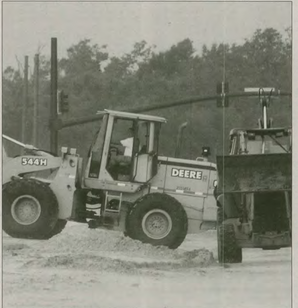
Mississippi Department of Transportation crews clear sand deposited by Hurricane Gustav in Gulfport Monday. Gustav hit the Gulf Coast weaker than expected, causing a drop in oil prices.
