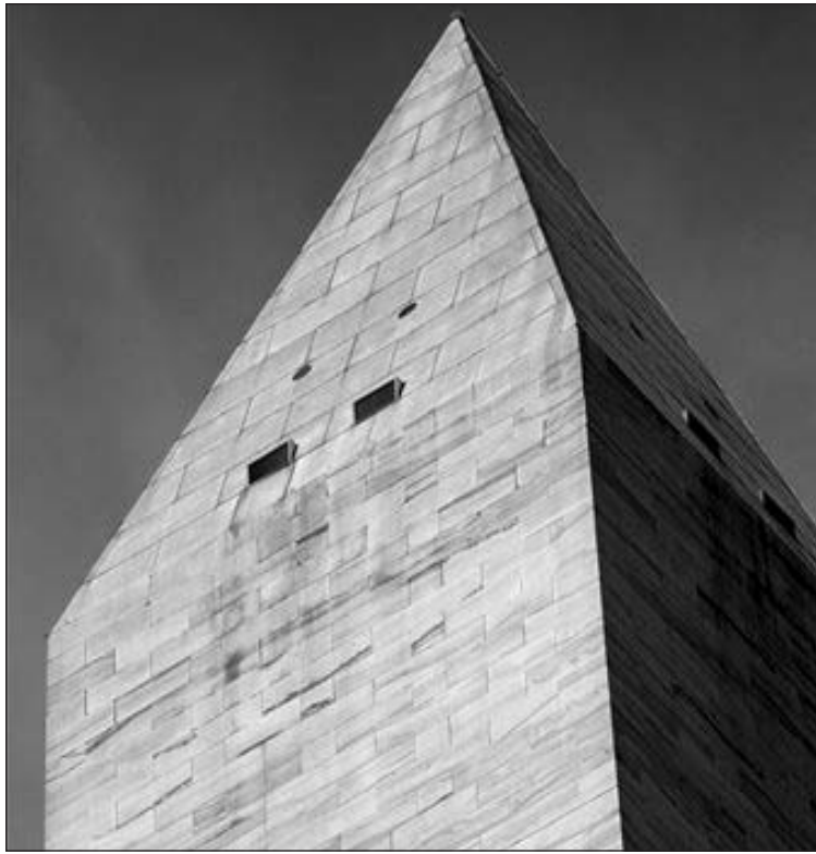
A 5.9 magnitude earthquake that struck the nation's capital Tuesday left a 4-inch crack in the Washington Monument.
