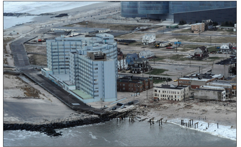
The Atlantic City boardwalk in New Jersey is washed away after Hurricane Sandy swept through the area Tuesday.
