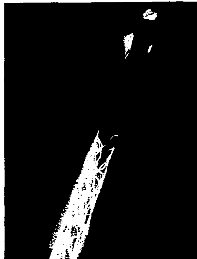
A discharge from the generator's ball to the ground taking place along one of the 22-foot supporting columns.
