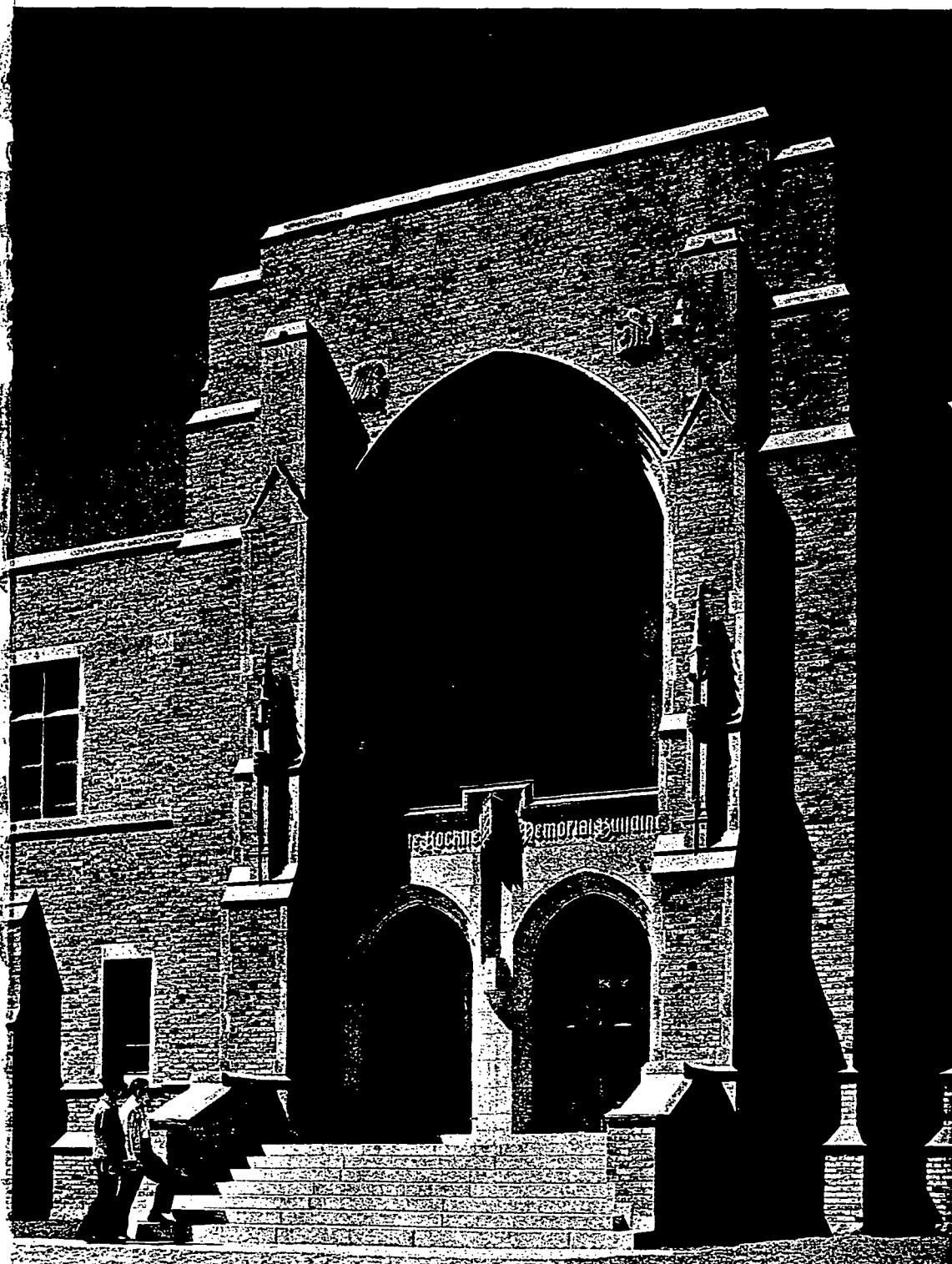
Main Entrance, Rockne Memorial Building
