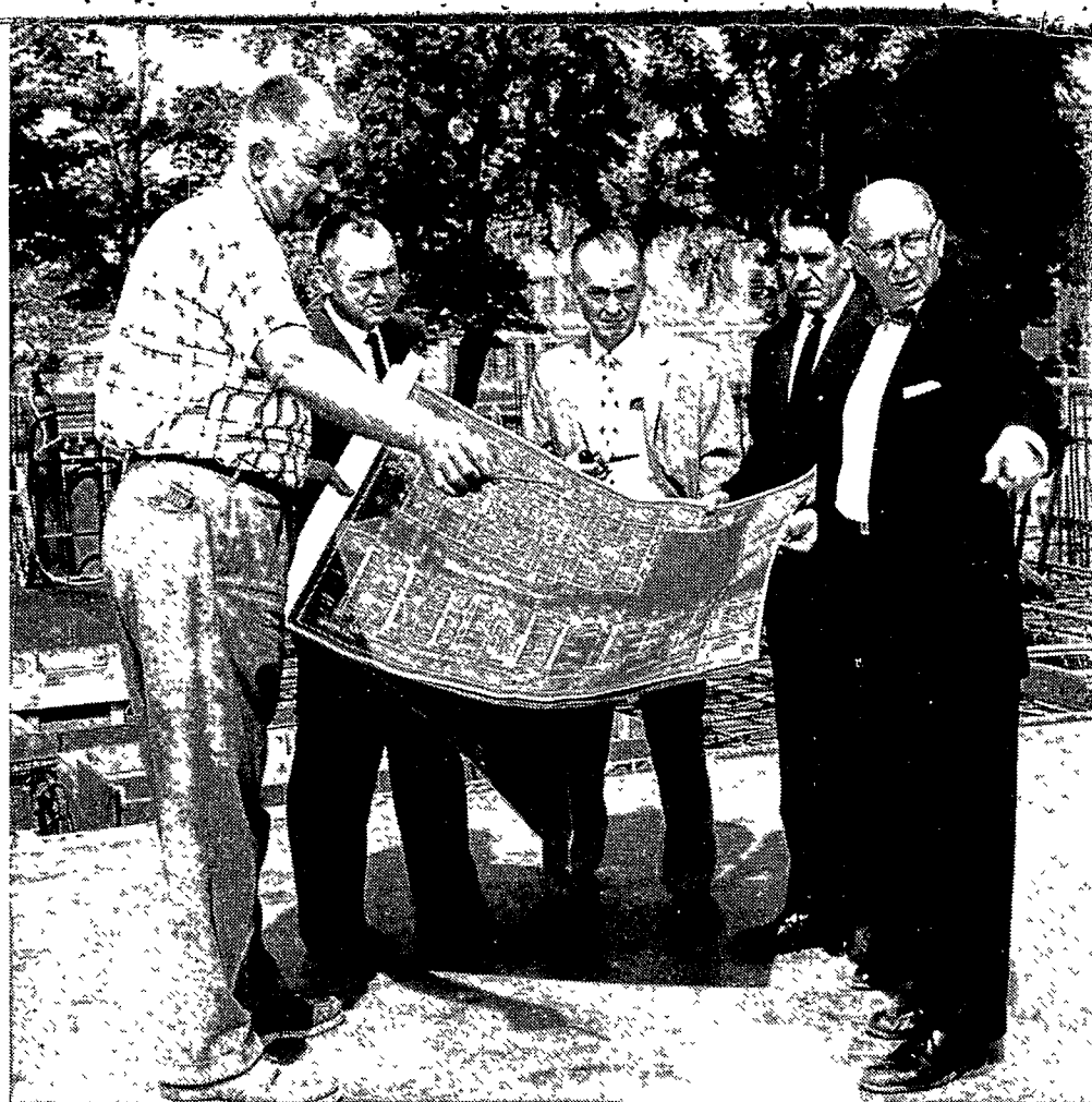
Charles Bennett, job superintendent, checks the blueprints for the new Radiation Laboratory with Messrs. Risser, Hamill, Magee, and Burton on the building foundation.
