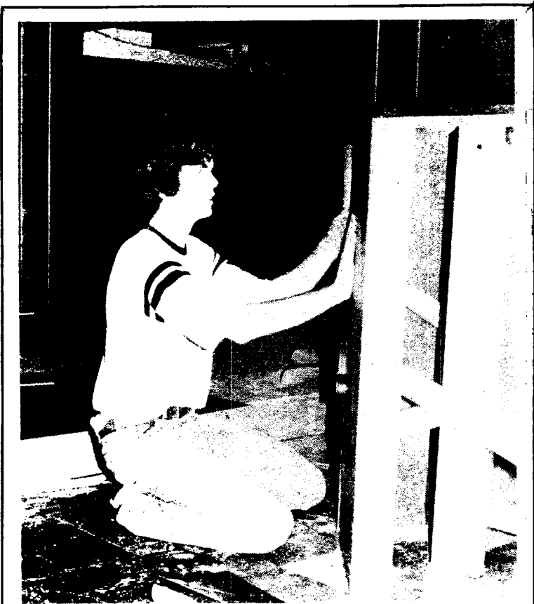
Construction currently underway in the LaFortune rathskellar is not part of the LaFortune renovation plan. With the Student Players production of "Come Blow Your Horn!" opening Thursday night, Mike Carlson (pictured here) and the rest of the stage crew are hard at work constructing the set. [Photo by Maureen Flynn]
