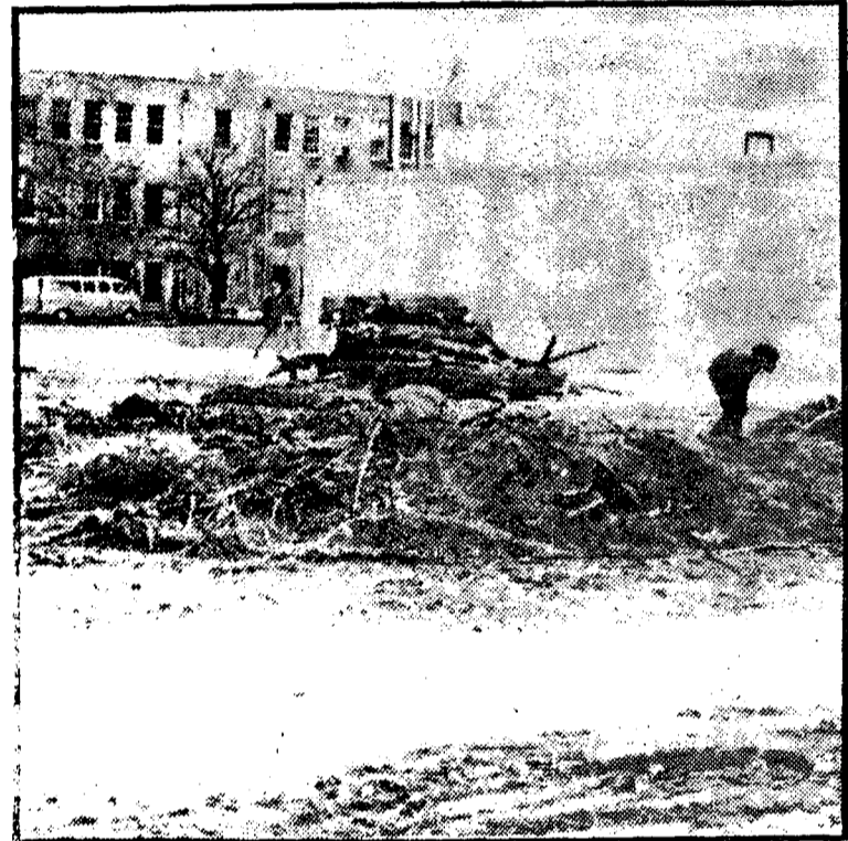
Trees are being removed as the construction of the Stepan Science Center gets underway. See related story on page 5. [Photos by Doug Christian].
