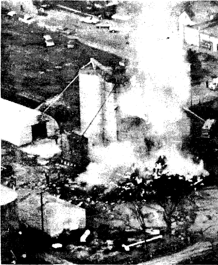
Firemen spray water on the flames of the Raymond, Nebr., Co-Op Grain Company elevator yesterday. The explosion on Tuesday left a total of four dead. The fire was fought through Tuesday night. (AP Photo)
