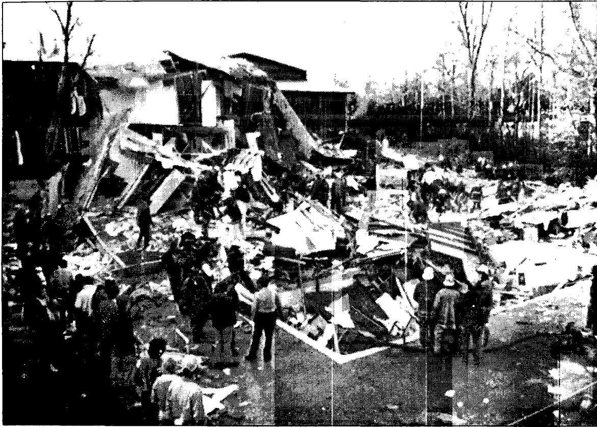
A set of six apartments at the Village Greene Apartment complex in Greenville, N.C., were leveled by a pre-dawn blast this morning, killing
