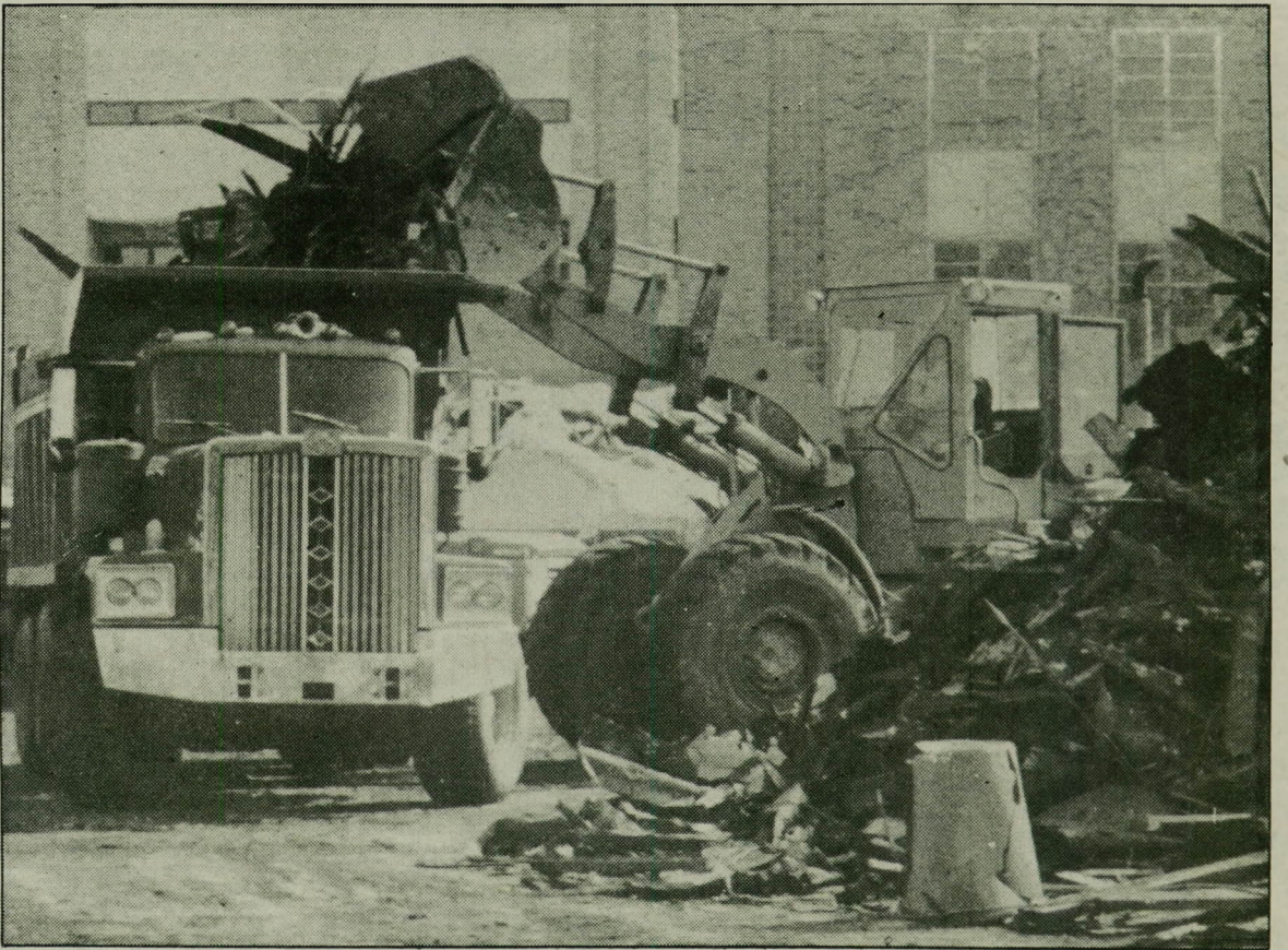
The recent snowfall has not stopped the tearing down of the Old Fieldhouse. Most of the historic building has already been torn down and has been carried off by dump trucks.
