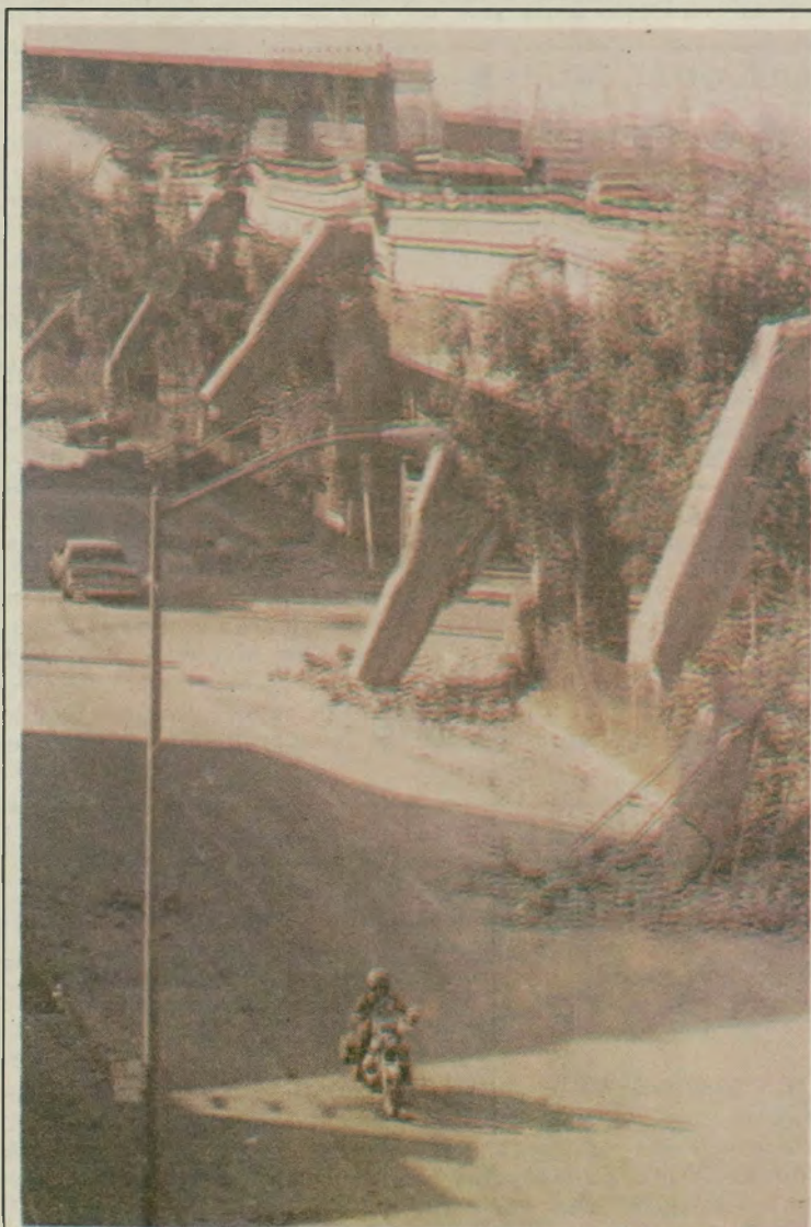
AP Photo A lone motorcyclist rides below the collapsed decks of the I-880 freeway in Oakland Wednesday morning. At least 200 are estimated dead from the collapse, which occurred when the Bay Area was hit by a 7.0 earthquake Tuesday.
