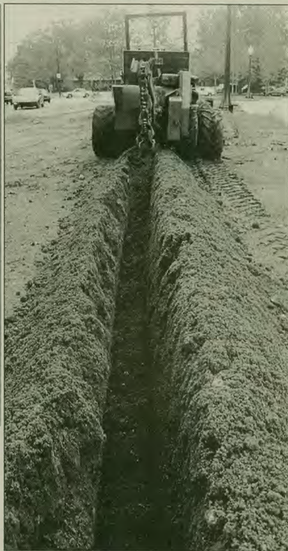
Tractors dug trenches as part of the new stadium's underground sprinkler system.
