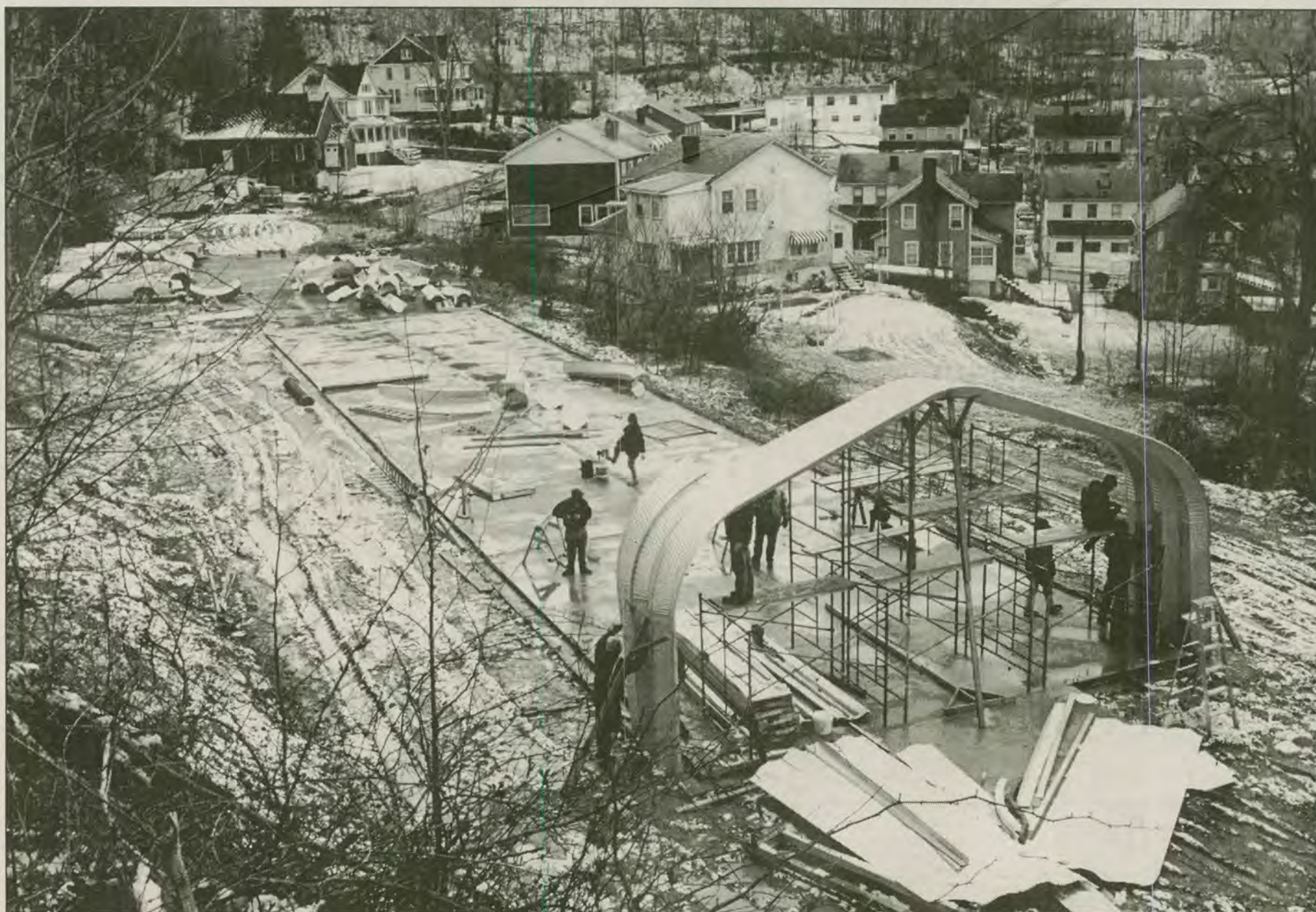
After dismantling the collapsed warehouse, the volunteers went to work putting it back together. The job was quite difficult; only three sections could be placed per day.
